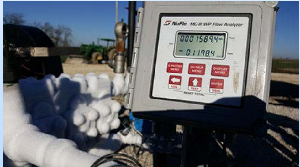
SCADA System installed on wells
